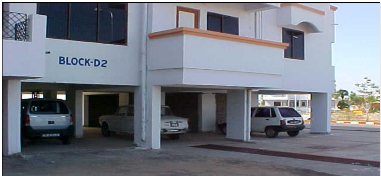
Figure 5: RC Frame Buildings with columns in open ground storey of 230mm width
