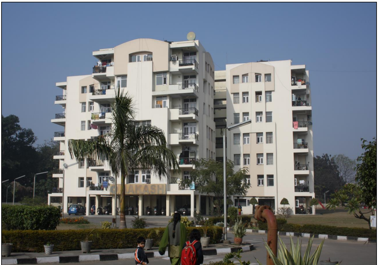
Figure 4: Typical RC Frame Buildings with Open Ground Storey
