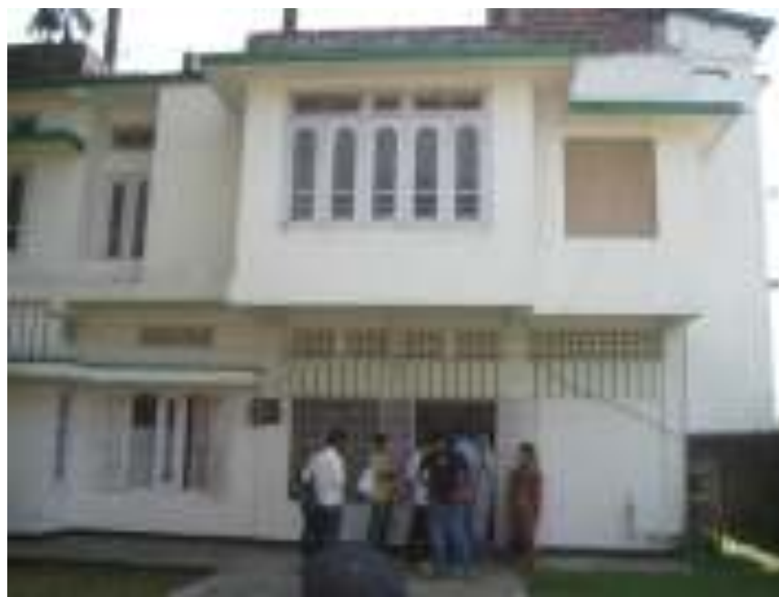
Reinforced concrete building
