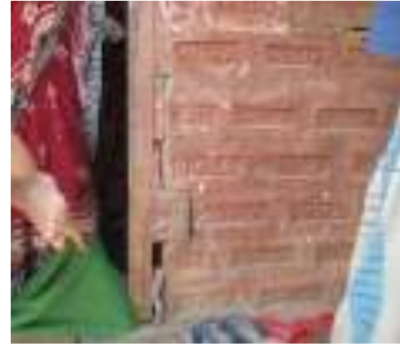
Brick Masonry Wall building
